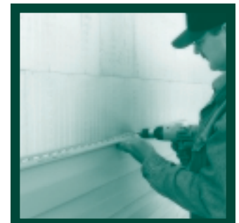
ICF homes can be built using conventional tools and methods.
