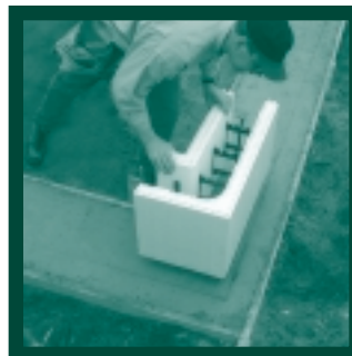
ICF walls are fast and easy to build
